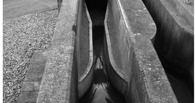
Venturi flume: BS3680 Part 4C / ISO 4359
